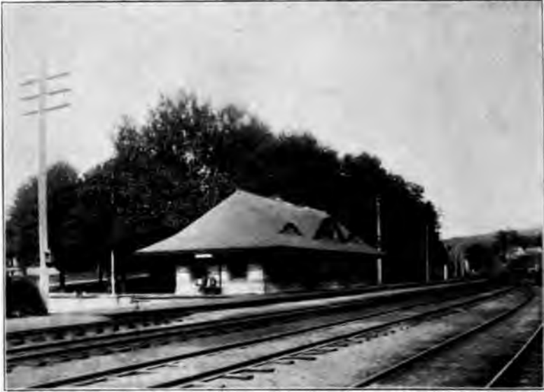
A MODEL WAY-STATION ON THE LINES OF THE BOSTON & ALBANY RAILROAD
